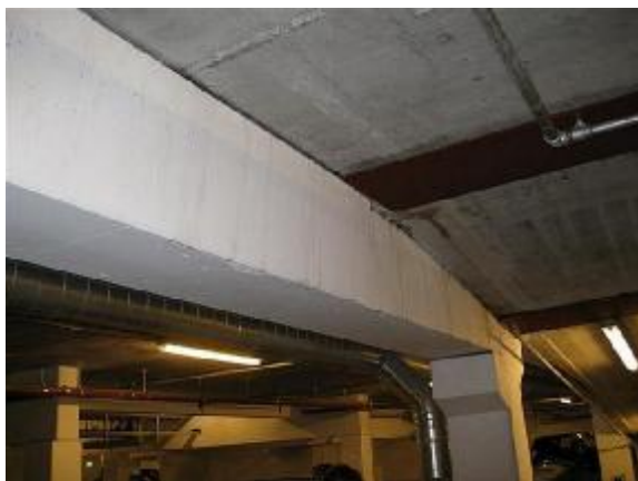
Underside rampe tv -1
